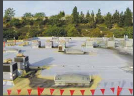
View of partially completed ccSPF installation
