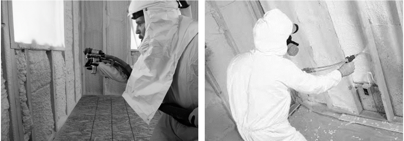
Figure 1: Visual of high pressure (left) and low pressure (right) products under study
