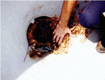
Remove debris from the roof system: Leaves and organic matter should be routinely removed from drains, scuppers, gutters, and the field of the roof.
