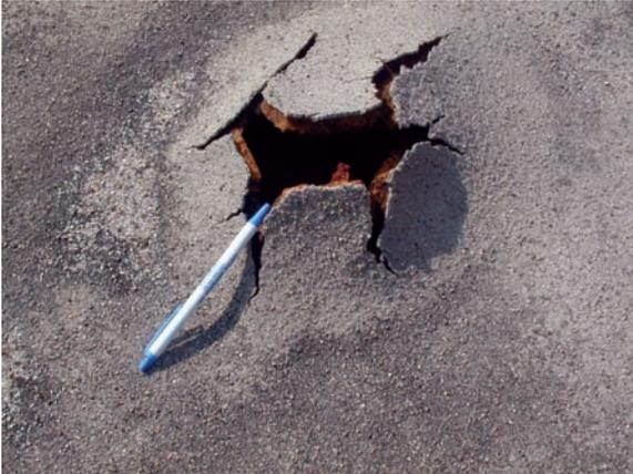
1. Thoroughly clean the roof surface around the damaged area of all dirt, dust or other contaminants with a rag and clean water. Allow to dry completely.
