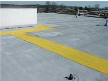
Minimize foot traffic to that necessary for the maintenance of the system or equipment. Walkways may be installed to help protect areas normally used by personnel. Check with manufacturers or contractors before installing.
