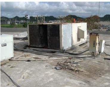
The roof should not be used for storage of HVAC repair parts, lumber, signs or any other unnecessary equipment.
