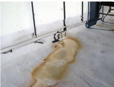
Prevent damage to the roof system from exposure to harmful chemicals or substances. Vents should not exhaust harmful materials onto the roof surface. HVAC condensate should not be drained onto the roof.
