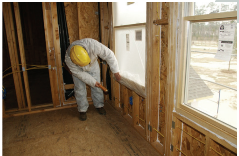
Figure 10: Sealing the windows
