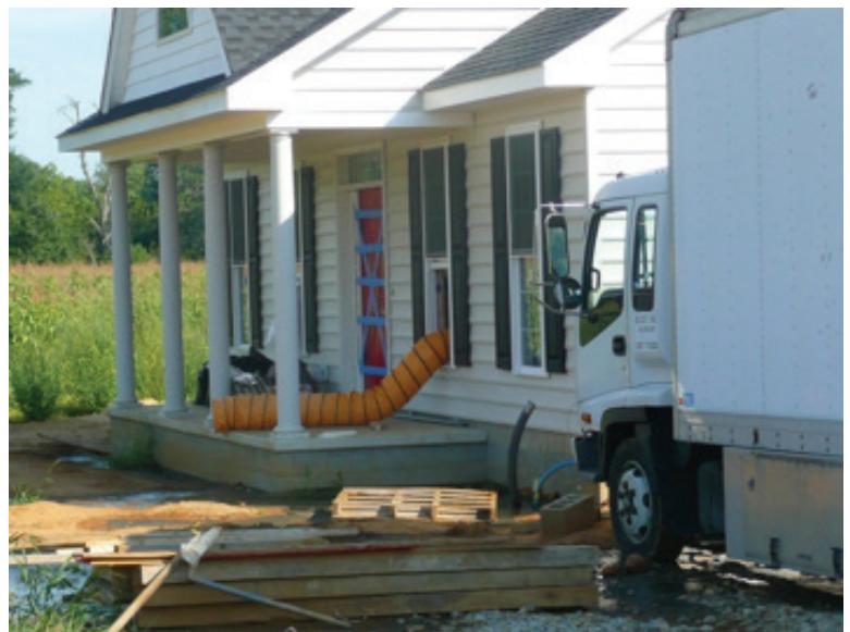
Figure 12: Provide adequate ventilation
