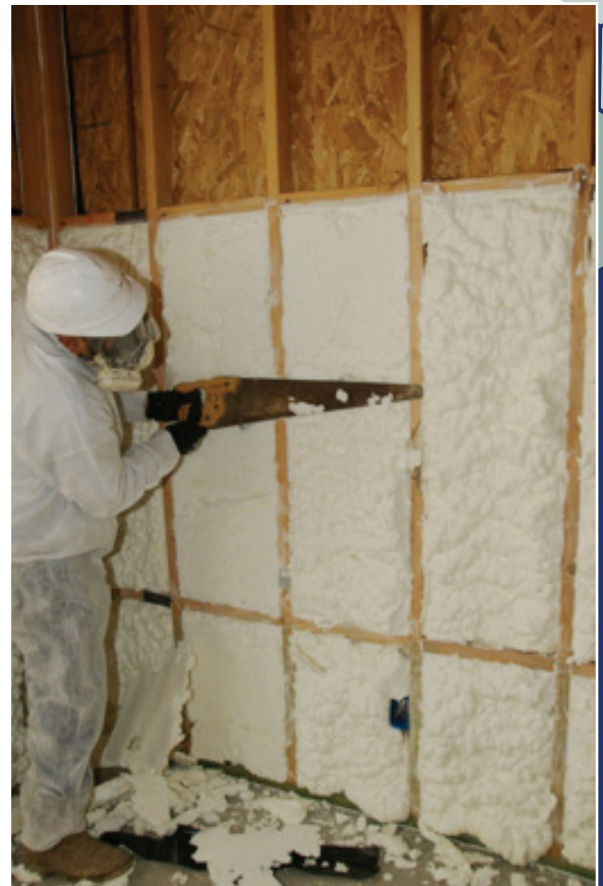
Figure 15: Contractor trimming foam
