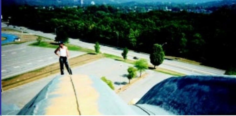
The University of West Virginia chose SPF for the 174,000 sq. ft. roof of the Evansdale Coliseum (above, cover). The SPF roof was installed in 1975 and recoated in 1991.
