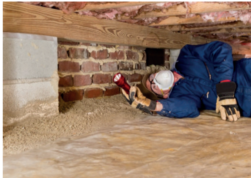
FIGURE 3. Visual termite inspection
