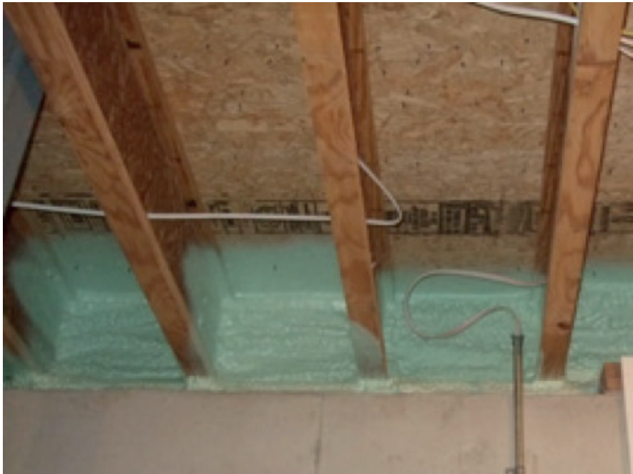
FIGURE 12. Closed-cell SPF insulation at the foundation-framing area
