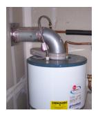
Figure 3: Direct Vent water heater. Sealed-combustion appliances are located close to an outside wall and vent through the wall. A double-walled vent tube functions as both air intake and exhaust flue. (No special requirements when air sealing building.)
