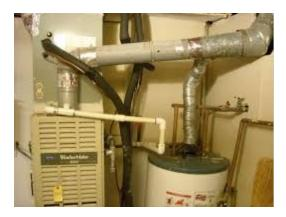
Figure 2: Typical open-combustion furnace co-vented with open-combustion water heater. (Requires fresh air source.)
