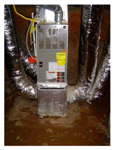
Figure 5: Draft fan-assisted HVAC system in a crawl space. The fan is designed to pull combustion by-products out of the heat exchanger and direct them into the exhaust flue. The fan does not propel the exhaust gases up the chimney; these appliances rely on the bouyancy of the hot exhaust to rise up the flue and vent out. This appliance is open-combustion and subject to the aforementioned considerations.
