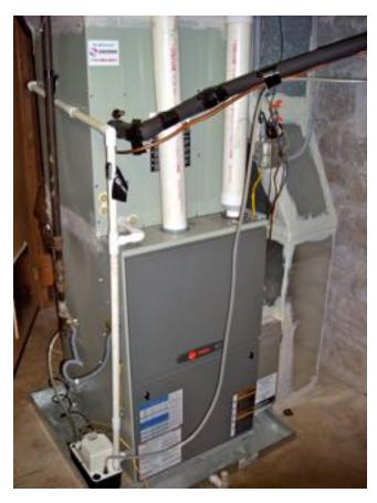
Figure 6: Typical sealed-combustion HVAC system. Air supply and exhaust is through the PVC piping. (No special requirements when air sealing building.)
