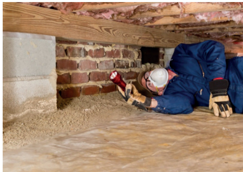
FIGURE 3. Visual termite inspection
