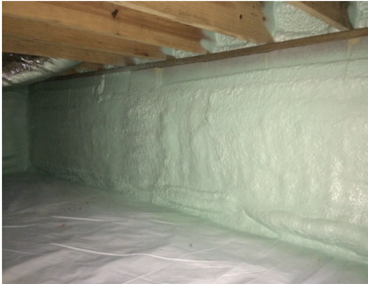
FIGURE 16. Installation of SPF to provide termite inspection strip
