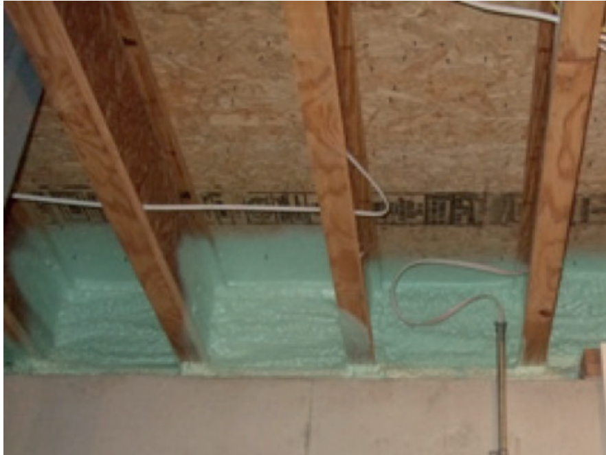
FIGURE 12. Closed-cell SPF insulation at the foundation-framing area
