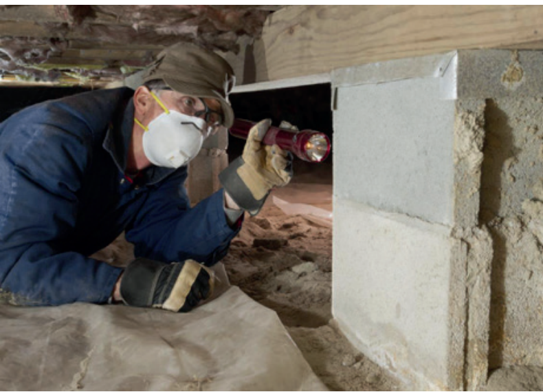
FIGURE 3. Visual termite inspection
