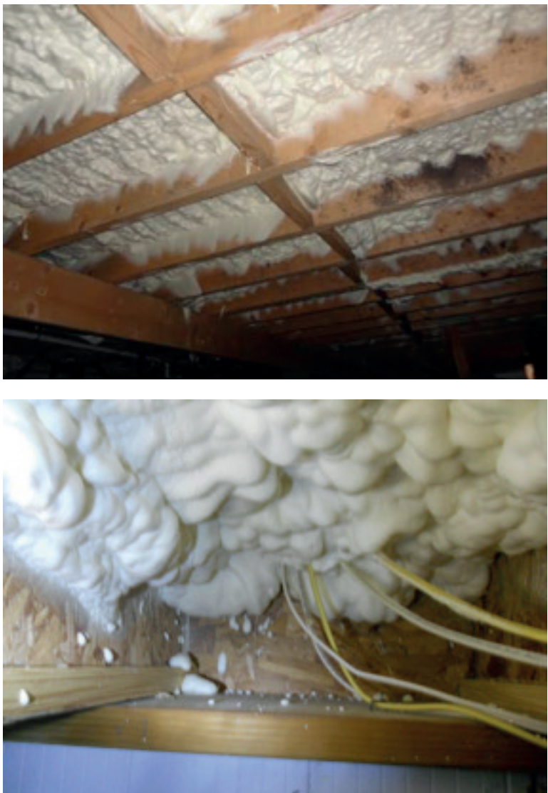
FIGURE 17. Installation of SPF below the subfloor allows complete access to the band joist and sill plate for inspection.
