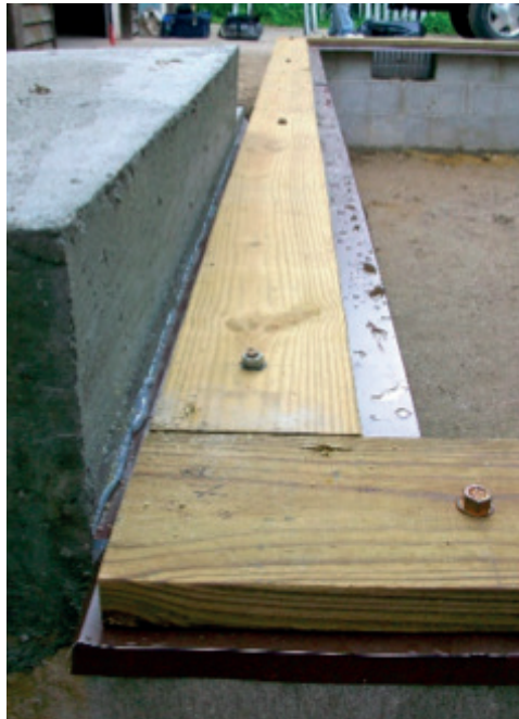
FIGURE 10. Physical termite barriers and shields
