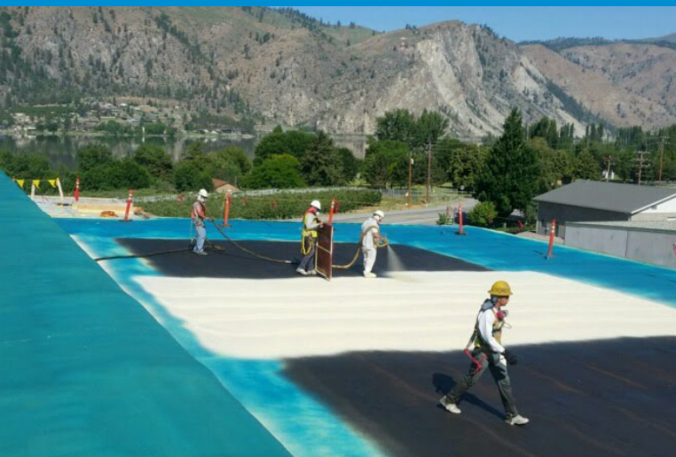
Auvil Fruit Company - Ultra-Thane 230 Spray Polyurethane Foam System Over Cold Storage
