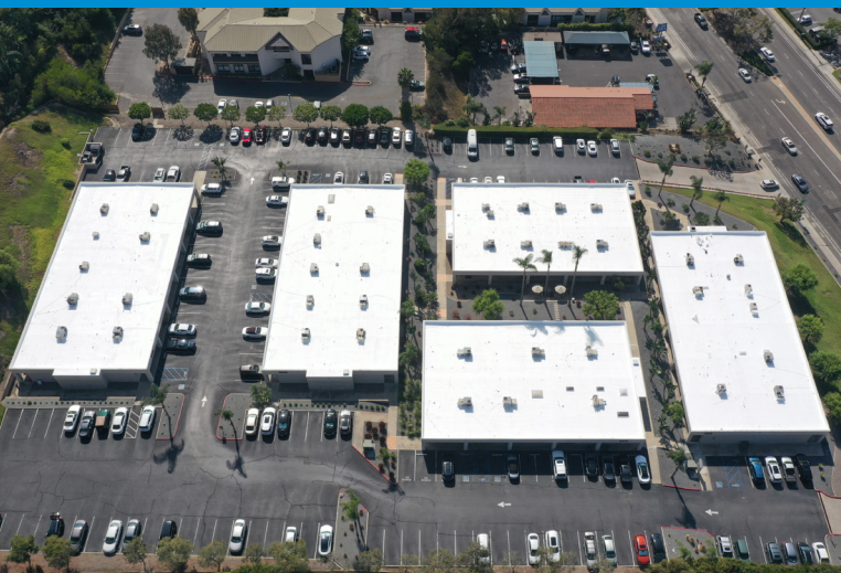
Encinitas, CA Properties - Ultra-Flex 1000 Acrylic Coating for Roof Restoration
